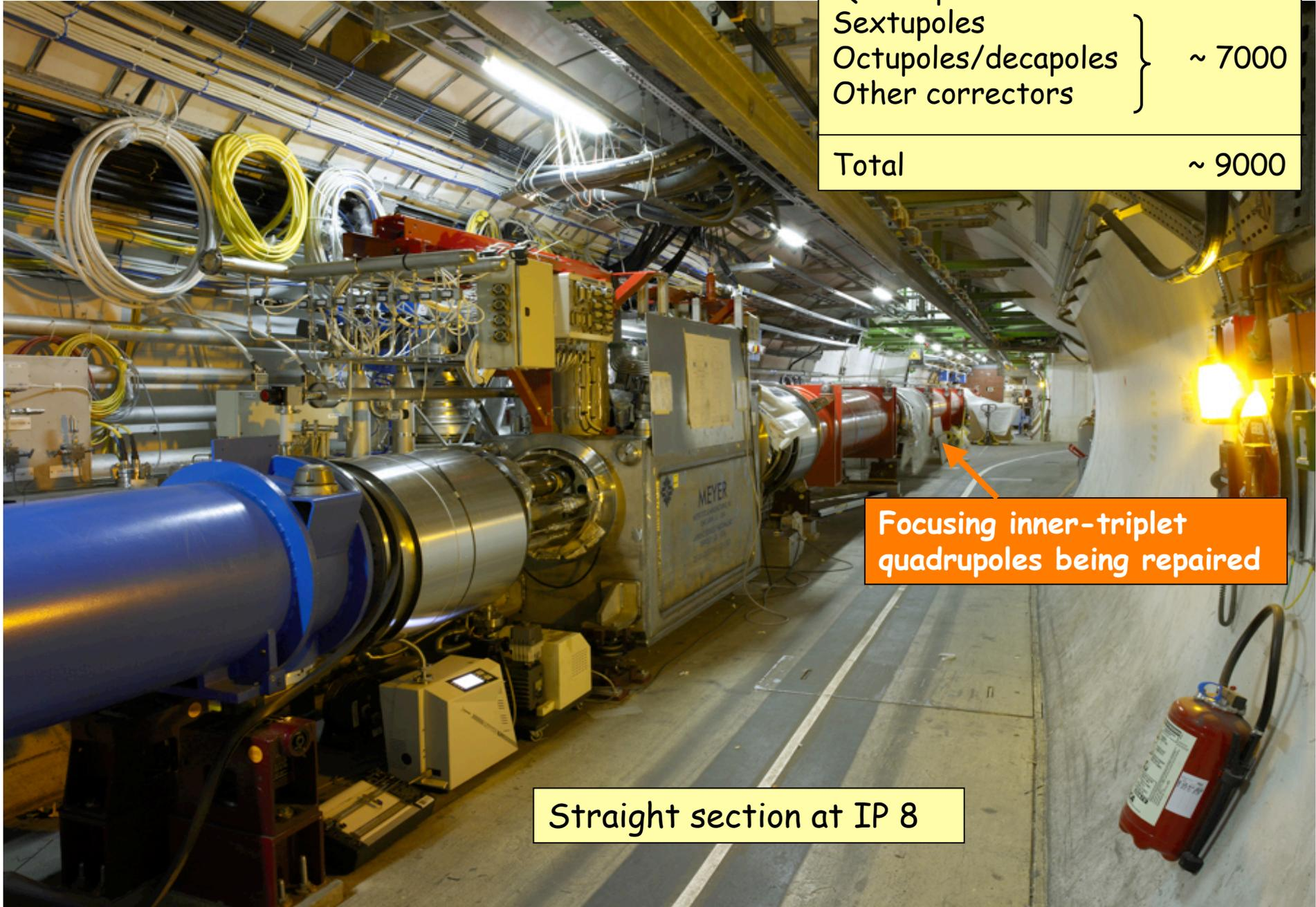
Focusing inner-triplet quadrupoles being repaired
